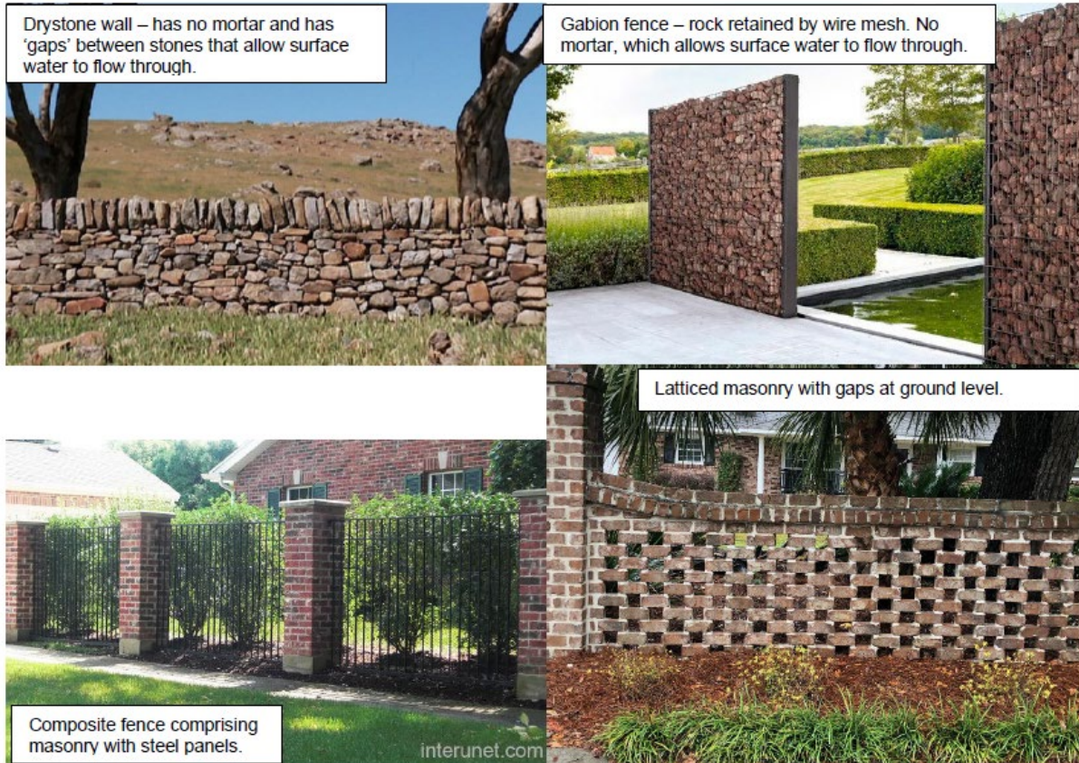
Figure 3 Mr Paul’s masonry fence examples
